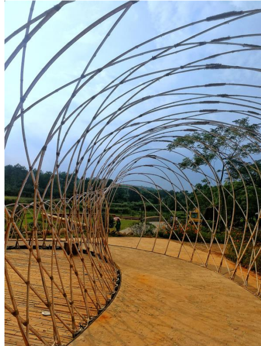
Figure 2. Bamboo structure compiled according to elastic line and geodesic line. By Feng Deng.
